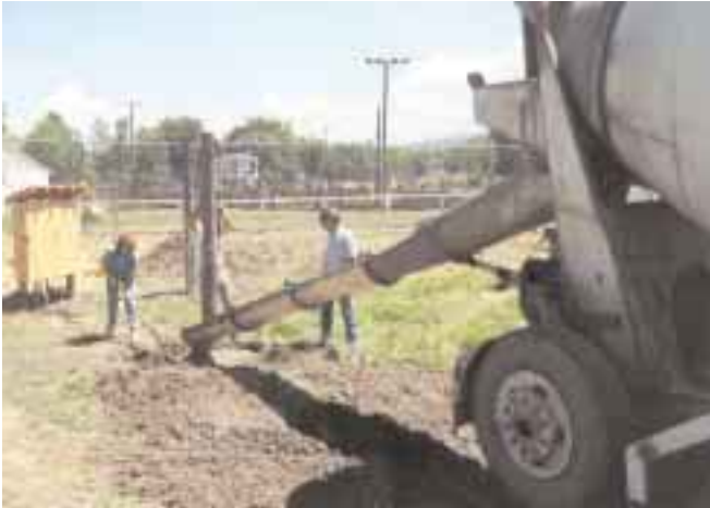
All the concrete work was done prior to the workshop.
