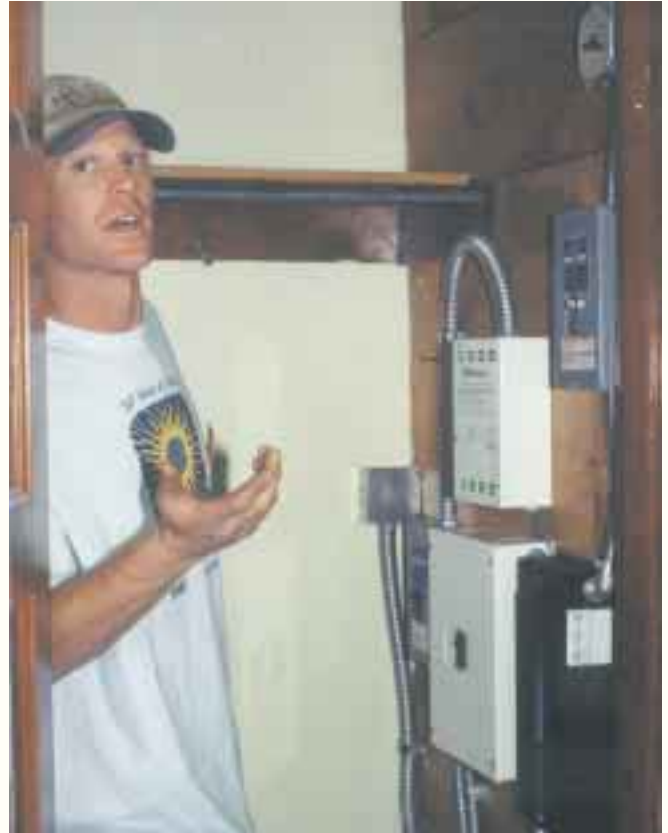
Co-instructor Joe Schwartz explains the finished power wall in the EORenew office closet.
